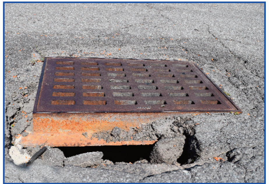
The parking lot at NFHS is 20 years old and needs repair.
